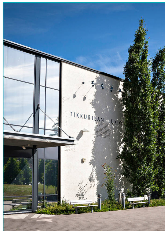
Tikkurila School, modernised as part of the ESCO project.
